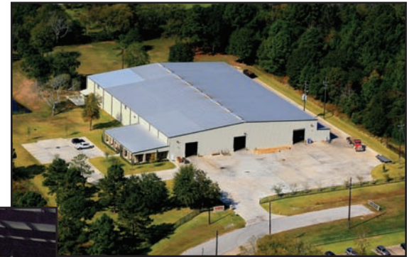
Vulcan Finned Tubes handles all emergency situations from its 50,000-square-foot facility that sits on five acres in Tomball, Texas.
